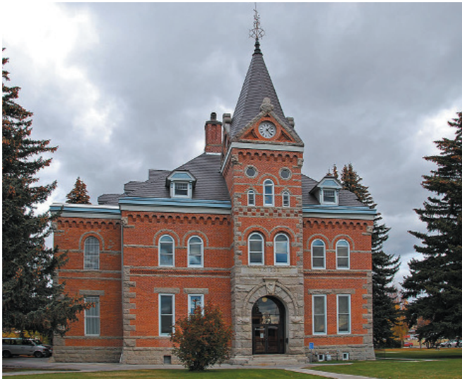
Jefferson County Courthouse in Boulder, Montana
